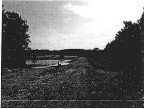
D-1778 Sherrill Pond Dam
